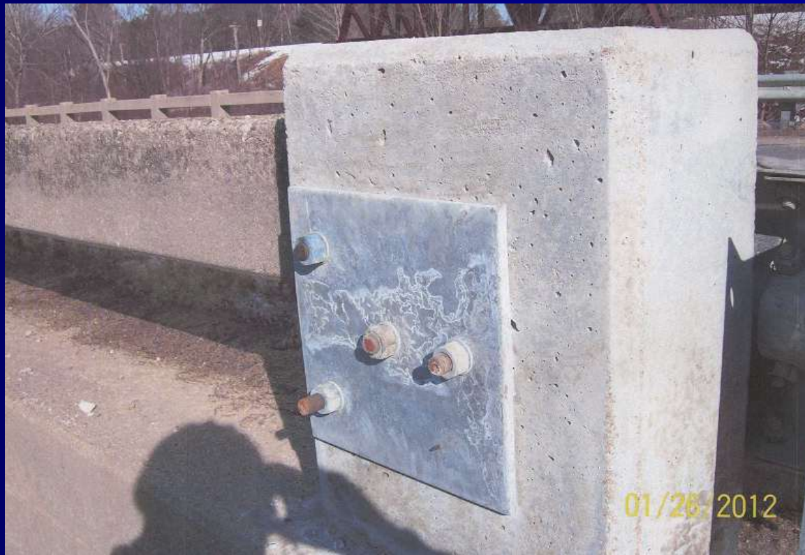
Back Side of Repair
