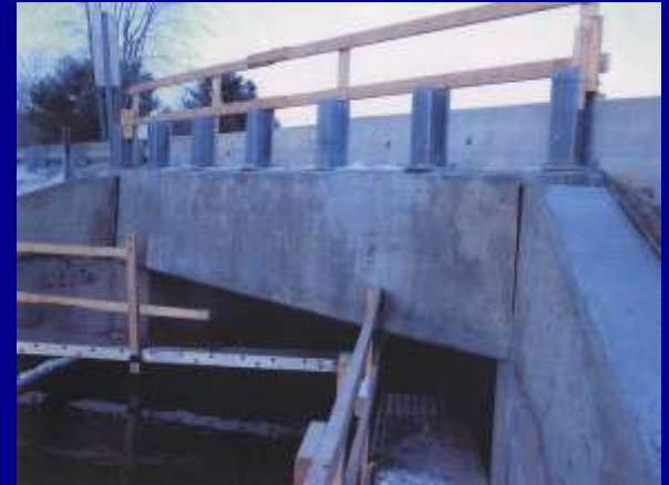
Example of Safety Rail being used
