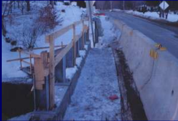
Stub Post during Construction
